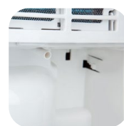
condensate drain hole
